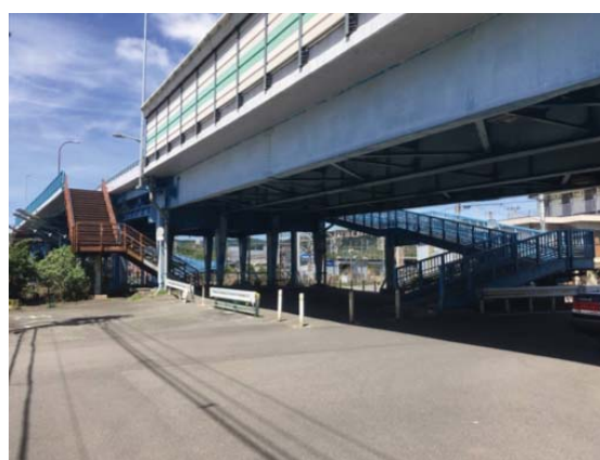
(b) under the footbridge
